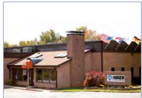
Hager Worldwide Corporate Office Hickory, North Carolina
